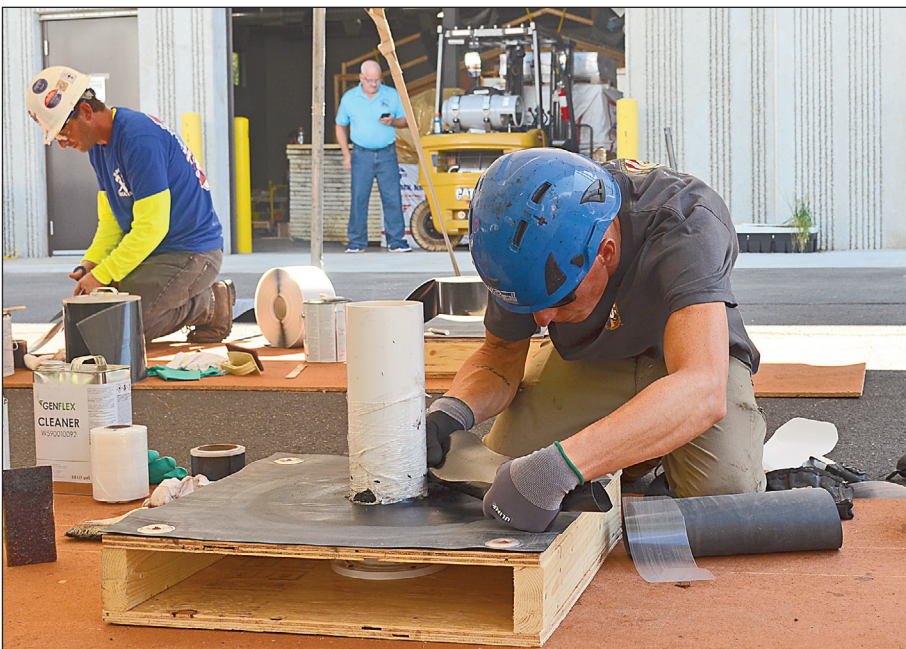
Roofers apprentices compete in "Best of the Midwest" at Local 96's training center.
